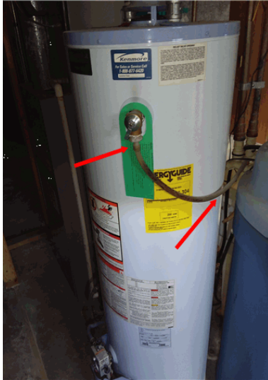
Tpr valve will not drain properly
